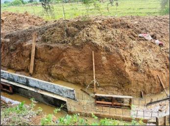
During the visit, canal construction was ongoing but temporarily stopped due to rain. It was observed that the canal level is currently lower than the paddy field level. The contractor plans to use burrow soil to raise the level to match the surrounding fields. The Farmers' Organization (FO) has requested burrow soil for leveling their paddy fields.
